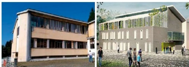
Figure 2 – The retrofitting intervention: building as is (left) and post-intervention (right)
