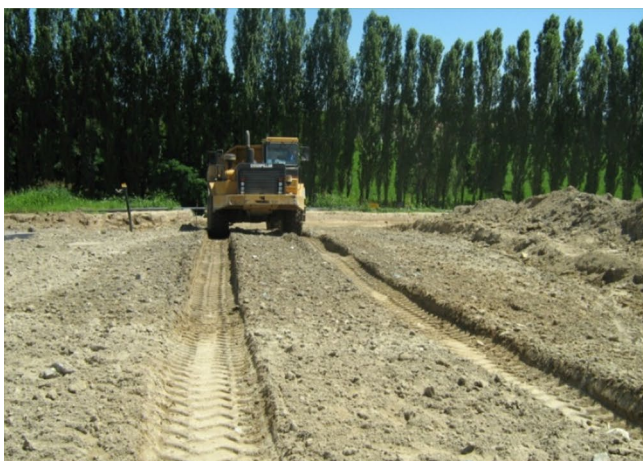
Fig. 9 Compaction of liner by dumper
