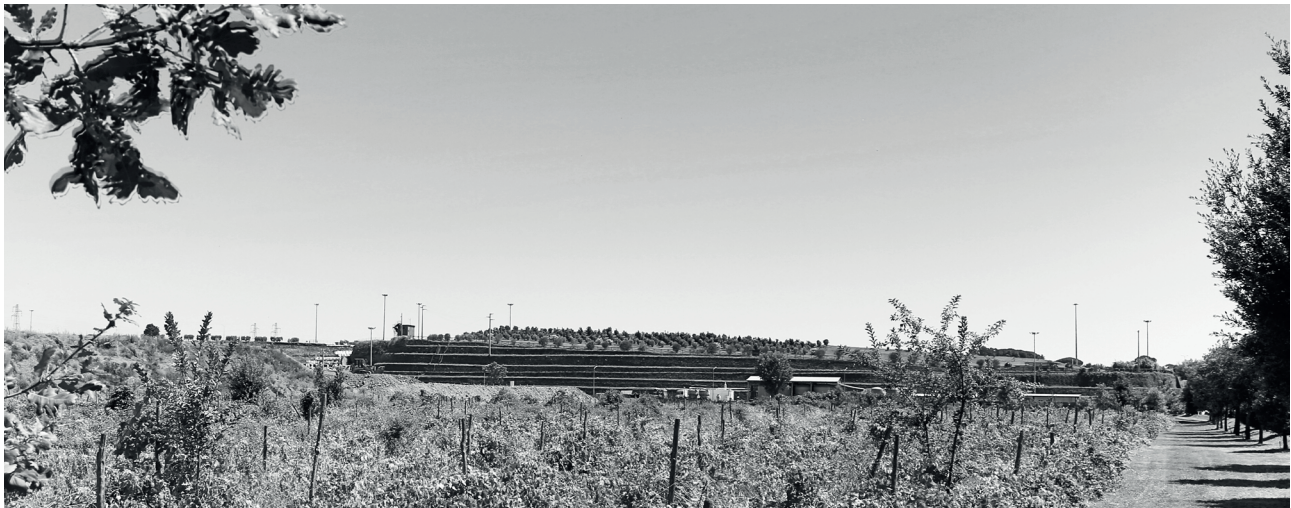
View of the existing landfill
