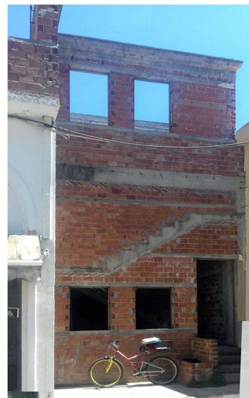
Fig.4 – Greek building stock: infill masonry in solid/hollow bricks 1
