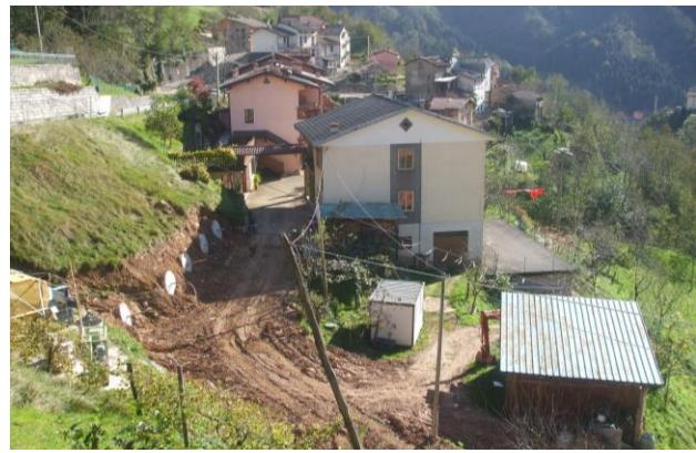
Figure 5. Installation of composite anchors at Cischele landslide (2014): (a) Bar and strands already infixed; (b) External concrete plates of alignment B visible at the ground surface near the house and below the road.
