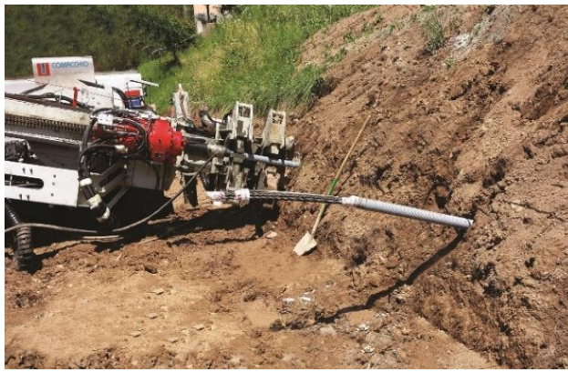
Figure 5. Installation of composite anchors at Cischele landslide (2014): (a) Bar and strands already infixed; (b) External concrete plates of alignment B visible at the ground surface near the house and below the road.
