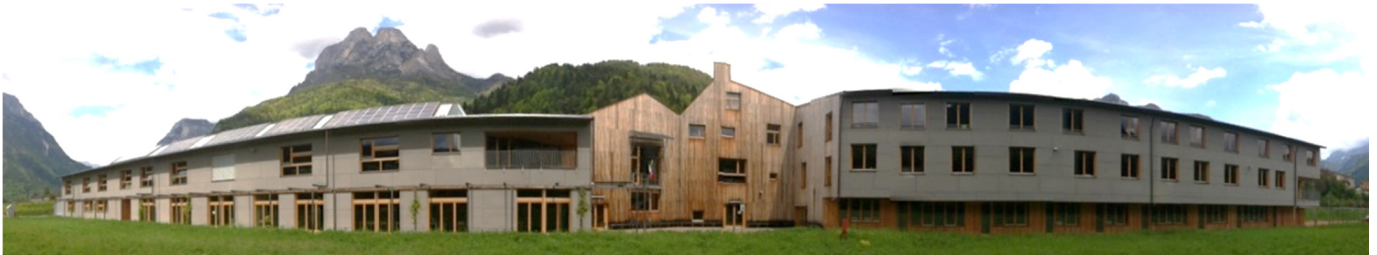
Figure 1. View of the school building in Agordo (from south).
