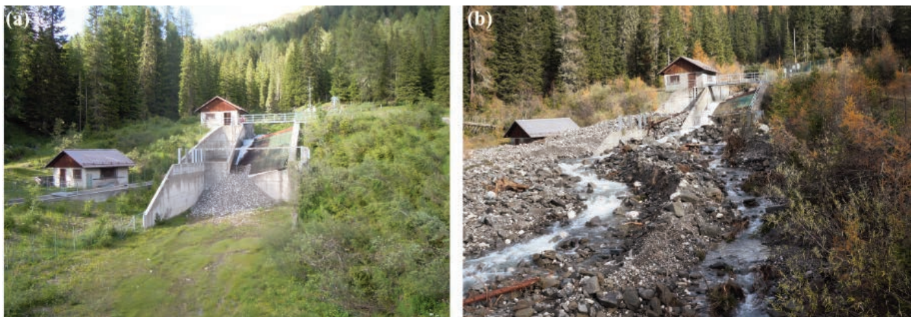
Figure 1. (a) Storage area of Rio Cordon monitoring station in August 2018 (pre-flood), (b) storage area in November 2018 (post-flood).
