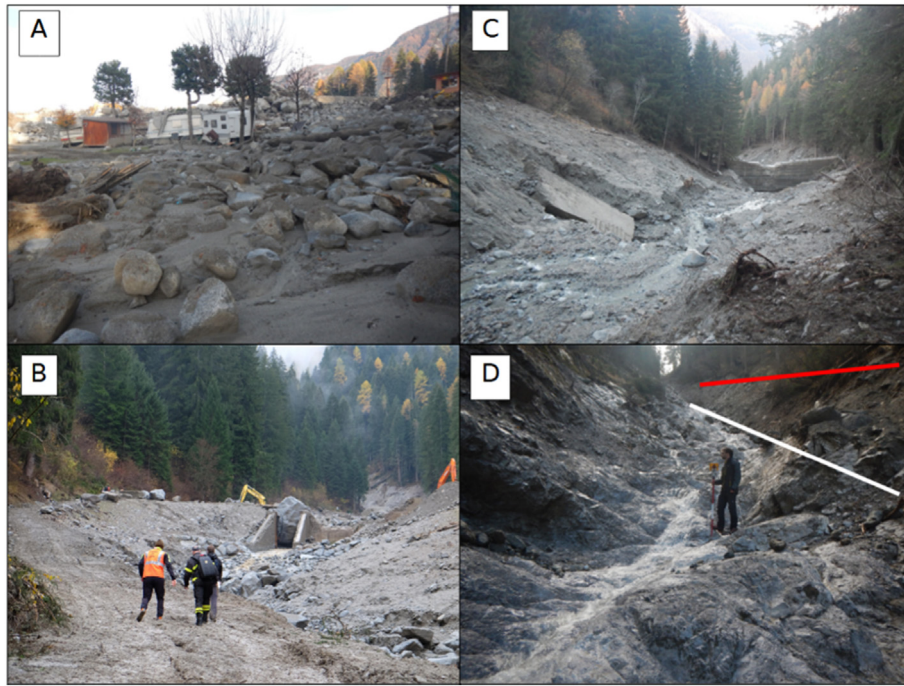
Fig. 2. Pictures of the post-event conditions. The debris deposit at the campsite (A), the sediment trap (B), the check dam channel reach (C) and the upper part of the channel (D); the white and red lines represent the minimum and maximum debris-flow front height with respect to the channel bed.
