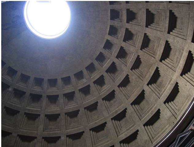
Fig. 4 – Interior of the Pantheon dome spanning 43 meters in diameter, with the oculus, the central hole having both a technical function (avoided closing the dome at the top) and an aesthetic purpose, 135 CE. (ArnoldDekker at Wikimedia Commons) Built in differentiated concrete, the dome remained unparalleled for more than 13 centuries.
