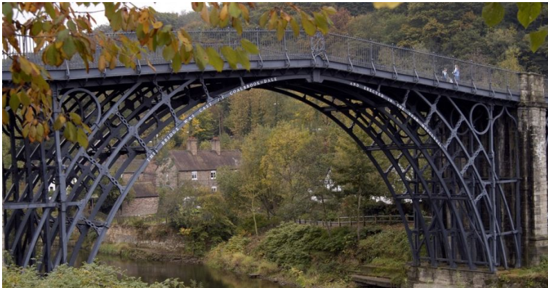
Fig. 6 – Cast iron bridge on the Severn at Ironbridge, England, erected by iron industrialists Abraham Darby III, John Wilkinson and others, 1781. (Wikimedia Commons) It was the first large iron structure ever built and demonstrated the potentials of cast iron obtained in large quantities and at relatively low cost with coke and puddling.
