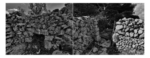
Figure 14: Dry stone details of the multicellular sheepfold of Dražica. Left: an entrance to the przgar through the škuja. Right: The dry stone walling is here done in a combined manner, the lower part constructed with double walls and the upper with a single wall, i.e., the 'Galloway wall' (2020).
