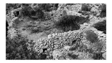
Figure 21: Details of the Ustrine commons older sheepfold: sheep passages (šku̇je) and the right partition wall fixed with capstones (2021)
