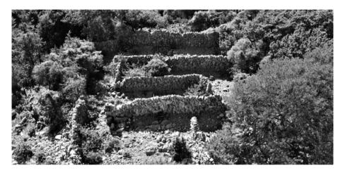
Figure 16: "This labyrinth-shaped sheepfold is mostly built of a single wall or in a 'Galloway wall' manner (2020).
