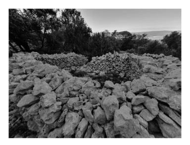
Figure 29: One of the sheepfold compartments; photo representing the massive double dry stone wall (2021)
