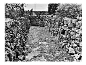
Figure 3: One of many small one-cell sheepfolds on the island of Cres, but with the distinction of the pavement with škrîji and a niche for tools (the environs of Osor [Mikaskegarine], 2021)
