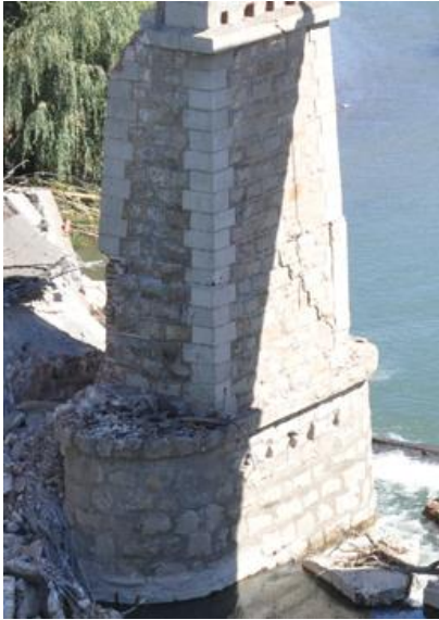
Figure 22 Claro River Bridge: diagonal cracks in a bridge pier [59].
