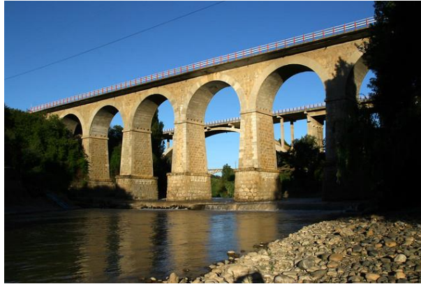
Figure 2 Image of the Claro River Bridge before the collapse
