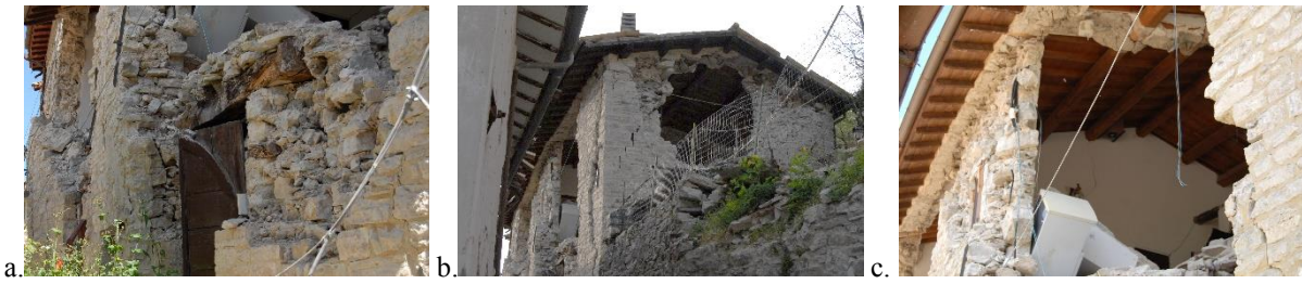
Figure 3: Examples of poor seismic behaviour in a strengthened masonry building, CSN: a) Not effective tie rods on bad quality masonry; b) overturning of last storey and c) of internal bearing walls due to r.c. curbs and to excess of stiffness and weight of reinforced timber roof
