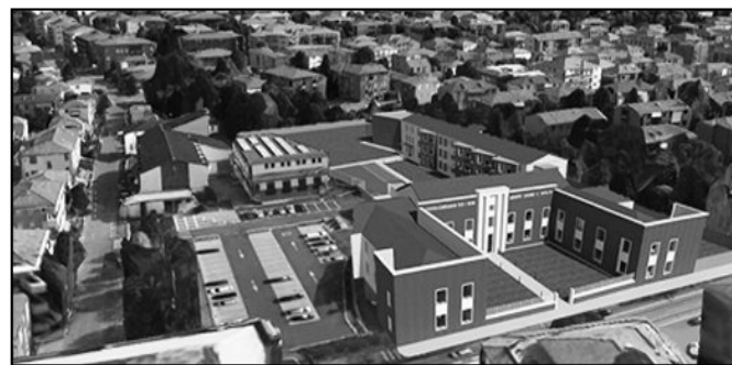
Figure 6 - Overview of the recovery project
