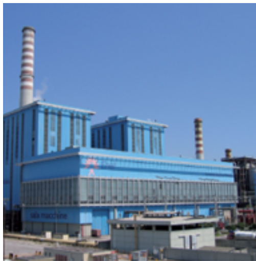
Figure 8-1. The "Andrea Palladio" plant at Fusina, owned by ENEL.
