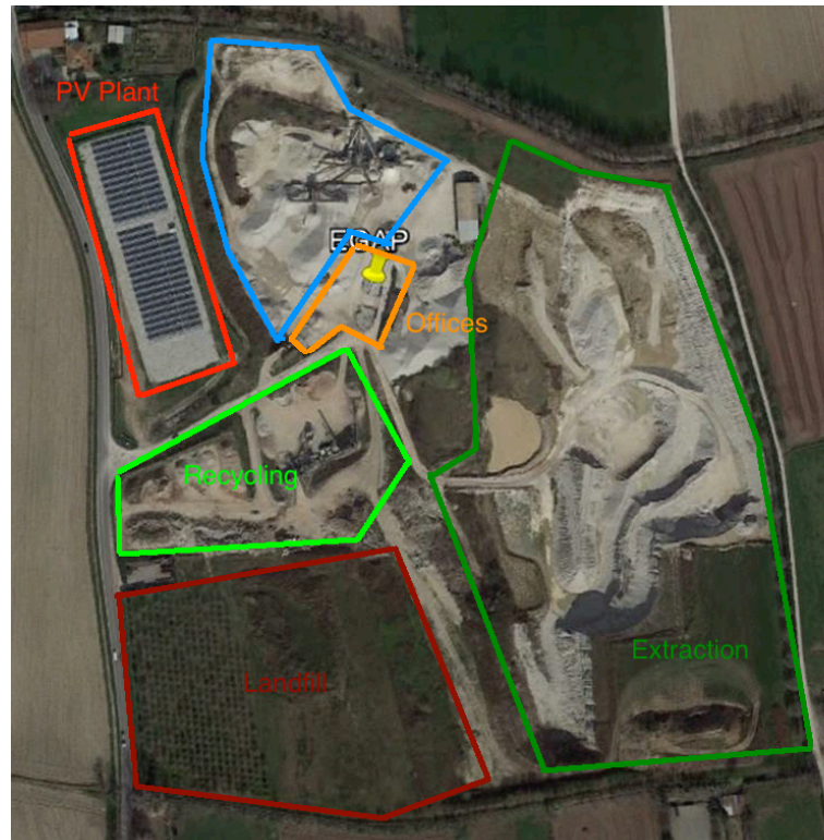
Figure 7-4. EGAP plant, Rosà (VI), Italy.
