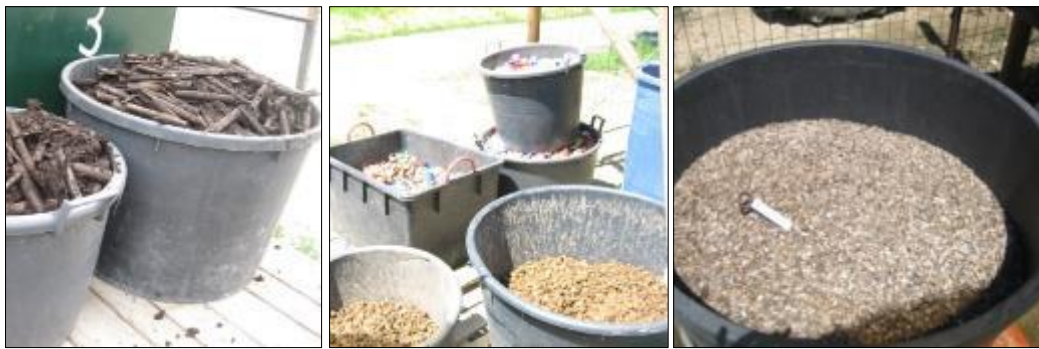
Figure 4.22 Emptying of the filters with separation of the substrates by depth level.
