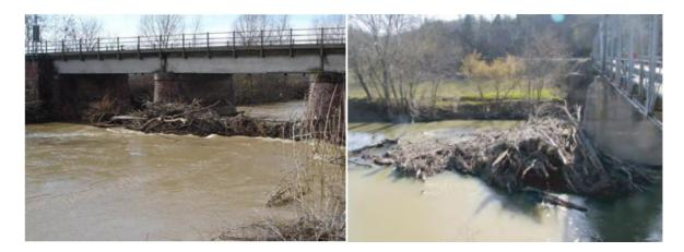
Figure 6: Hydraulic risks associated with large wood.
