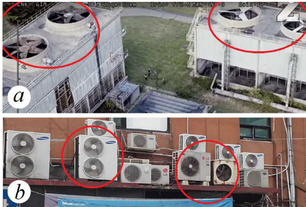
Figure 1: Use of different Fan Geometries for similar applications. Only one fan will feature the higher efficiency and, accordingly, the minimum electrical consumption and CO 2 emission.
