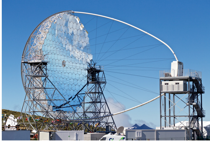
Figure 2.36: The current status (beginning 2019) of realization of the first LST telescope of the northern site in La Palma, Canary Island.
