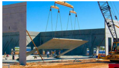
Figure 3.16: A tilt up building during its construction.
