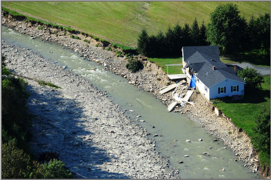
Figure 13: Impact of bank erosion on human properties.
