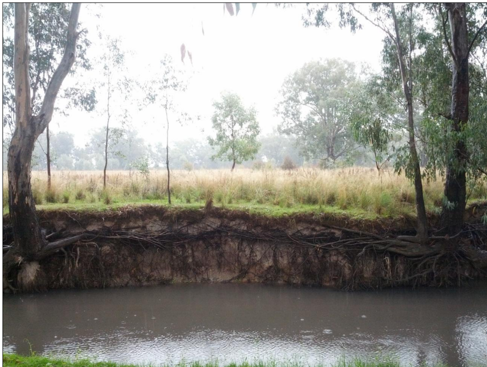
Figure 10: Stabilizing effect of riparian vegetation on the King River (Australia). Root plates, enhancing soil cohesion, contribute to reduce bank retreat.
