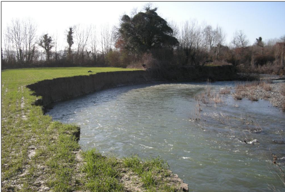
Figure 3: Large removal of soil by riverbank erosion.
