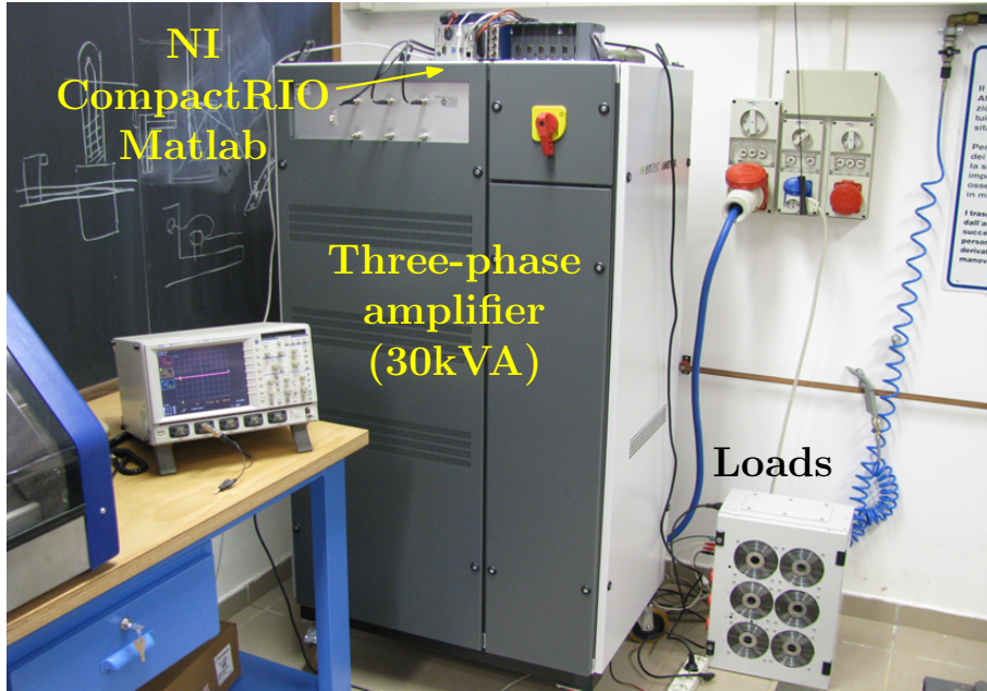
Figure 3.4: Three-phase experimental setup for load up to 30kVA.
