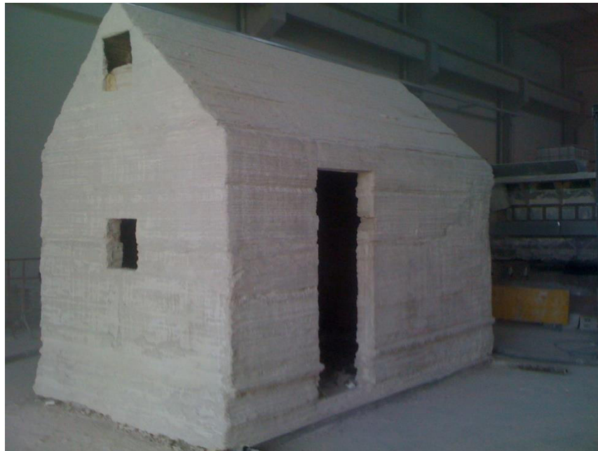
Figure 1.40. UnaCasaTuttaDiUnPezzo printed by D-Shape. [62]
