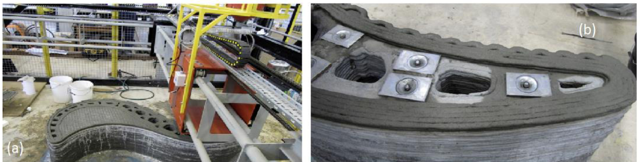
Figure 1.26. (a) the CP process; (b) detail of reinforced bench. [41]
