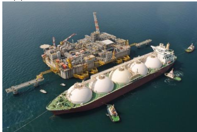
Figure 2.8 Off shore gravity based structures (GBS)
