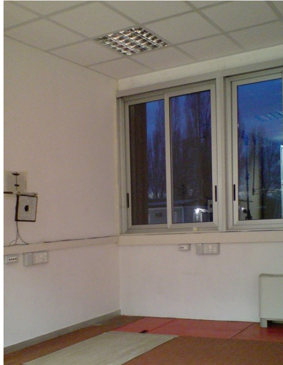
Figure 6.2: Image of the surveyed corner as seen by the thermal camera. The left wall is facing southwest and the right one is facing northwest. On the left wall are installed the thermal conductivity measurement apparatus and the air temperature thermographic reference.
