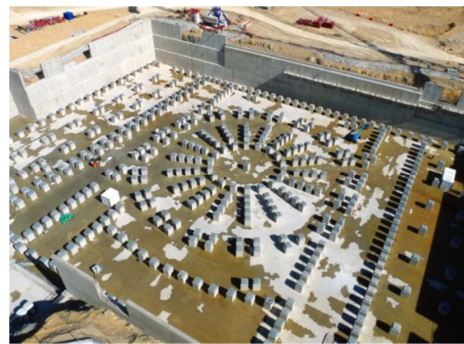
Figure 1-28: April 2012, completion of the antiseismic foundations of the Tokamak building
