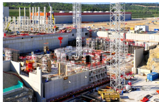
Figure 1-30: April-May 2015, state of construction of the Tokamak containment building
