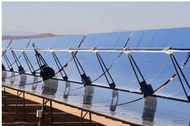
Figure 4.3. Parabolic trough system, example.
