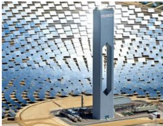
Figure 4.6. Solar tower, example.
