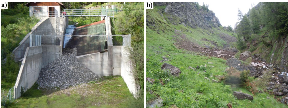
Figure 46: The bedload volume transported by the June 2014 event (a), the source area of the bedload event (b).
