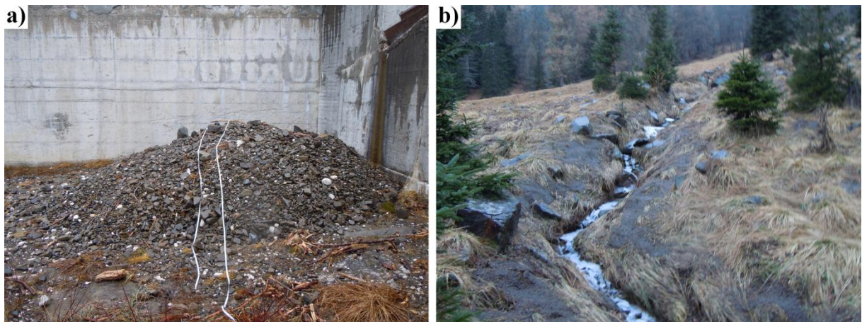
Figure 40: The bedload volume transported by the November 2012 event (a), field evidences along the debris flow channel (b).
