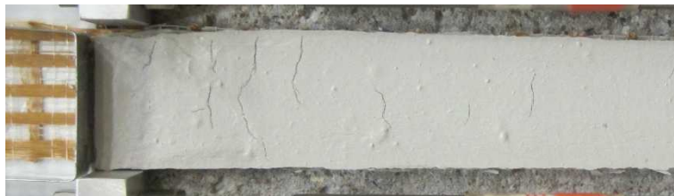
Figure 14. Shrinkage cracks on surface of specimen DS_330_43_2.
