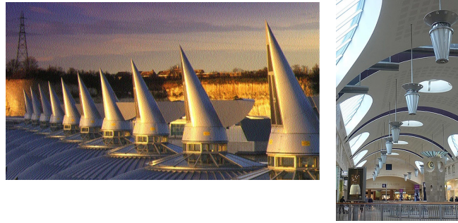
Figure 11 Wind scoops application on Blue Water shopping centre, Kent Source: http://www.battleccarthy.com/bluewater-shopping-centre-kent
