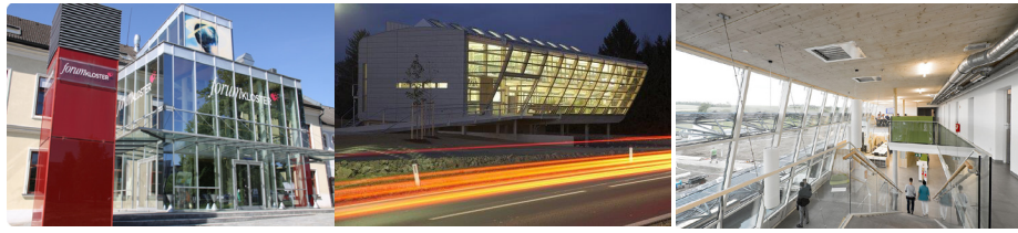
Figure 7 Examples of transitional spaces type b adopted into the mixed-mode solution. From left to right: Forum Kloster and Oststeiermarkhau (source: IEA EBC Annex 62 Ventilative Cooling International Ventilative Cooling Application Database [1.15]), Windkraft Simonsfeld AG (source: IEA EBC Annex 62 Ventilative Cooling International Ventilative Cooling Application Database [1.15])
