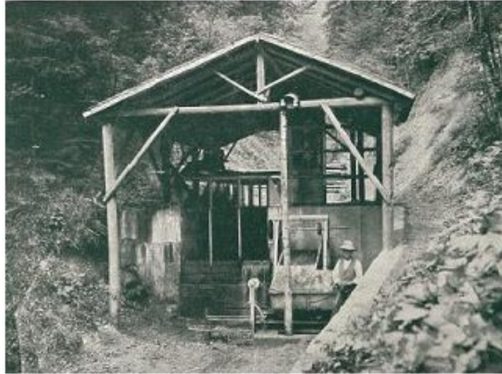
Figure 8: Initial Sperbelgraben runoff measuring station (after Engler, 1919).
