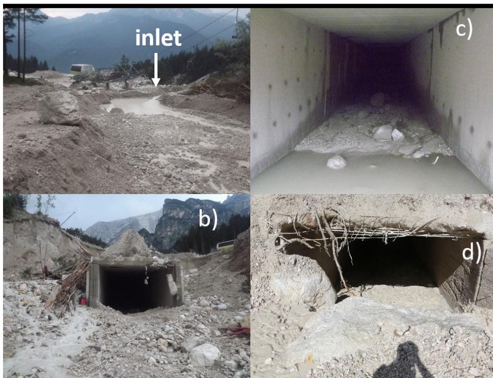
Fig. S5.2. Images of the culvert. Images of the inlet and exit of the culvert. Image a) the Ru Secco creek with the inlet submerged by deposits just after the event; b) inside the culvert close to the exit just after the event; c) the exit just after the event; d) the inlet during the sediment removal operations.
