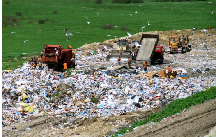
Figure 2.3. Problems of untreated landfills
