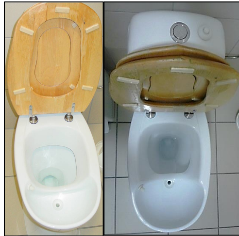
Figure 1.3. Toilet in flow separation
