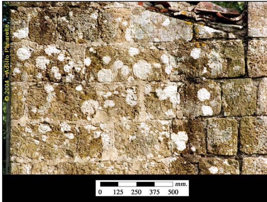
Fig. 6.3 - Lichens on the surface of an old building (Courtesy of Adolfo Panarello)
