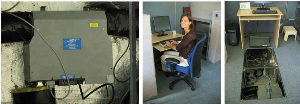
[Figures 2.45, 2.46: Personal Environmental Module (PEM) manufactured by Johnson Controls, Milwaukee, Wisconsin, connected to the workstation]
