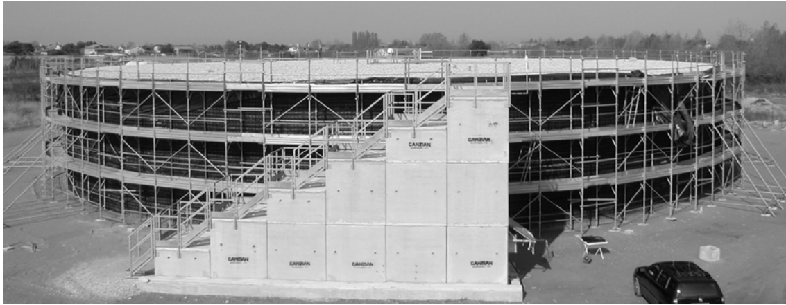
Figure 6.9: Treporti embankment at the end of completion
