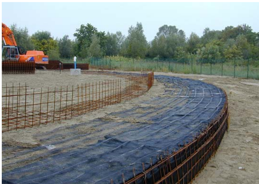
Figure 6.16: the first embankment layer with the geogrid
