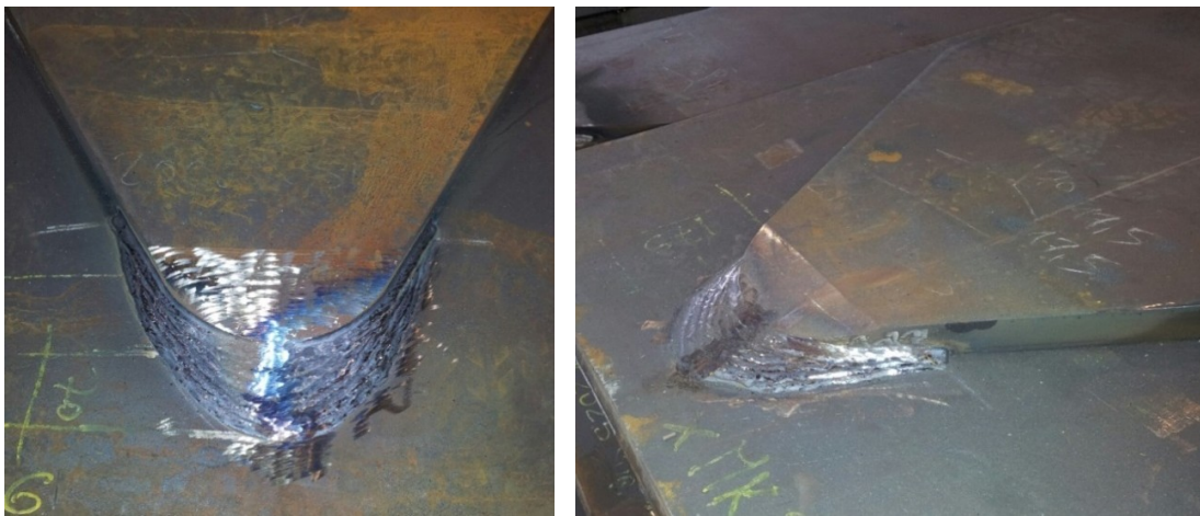
Figure 3.2. Example of practical design solution of a cover plate with pointed end.
