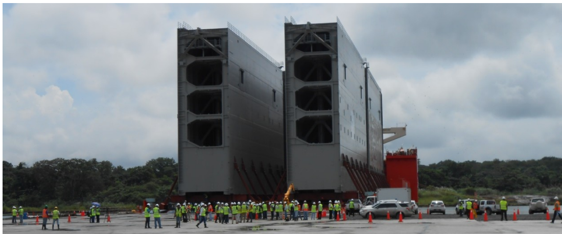
Figure 8.1. Some of the 16 lock gates at their arrival in Panama, after about 40 days of ocean traveling from Trieste (Italy).
