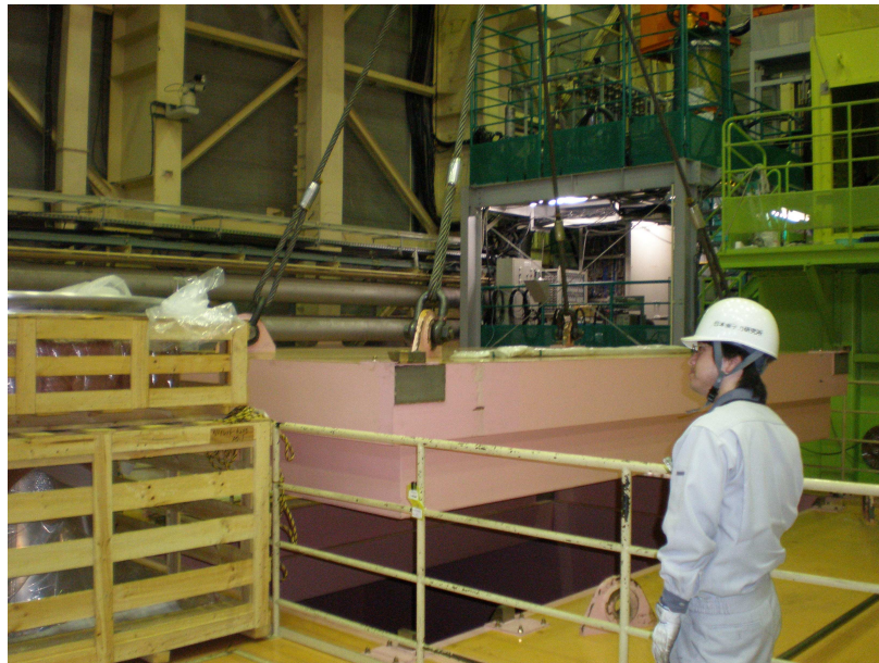
Figure 23 Removable top Concrete x-ray shield. Photo kindly supplied by JAEA NBI group.
