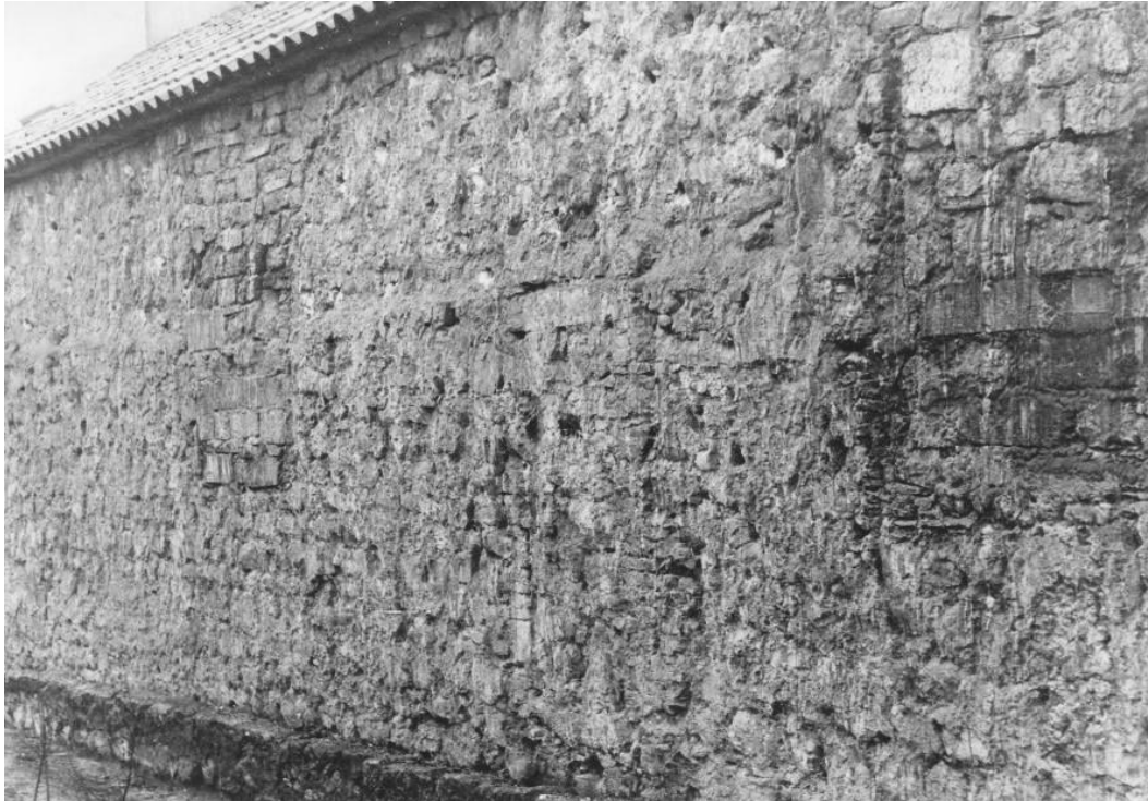
Figure 5.33: Northern wall of the church of St. Peter, older wall is visible protruding in the lower part (Archives of Conservation department in Rijeka, 1974)
