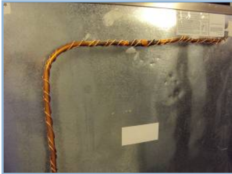
Figure 3.3.8 Suction line heat exchanger
