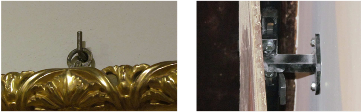
Figure 5.9 Examples of ordinary use of anchoring systems in the attachment of art objects to structural elements
