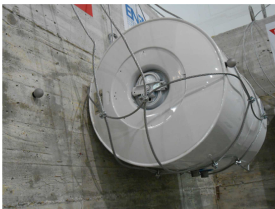
Figure 3.68 Anchorage of a water heater to concrete wall by means of two fixing points with A anchors and M10 steel stud
