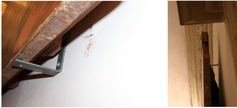
Figure 5.15 Ordinary fastening of art objects by means of plastic expansion anchor (left) and chemical anchor (right)
