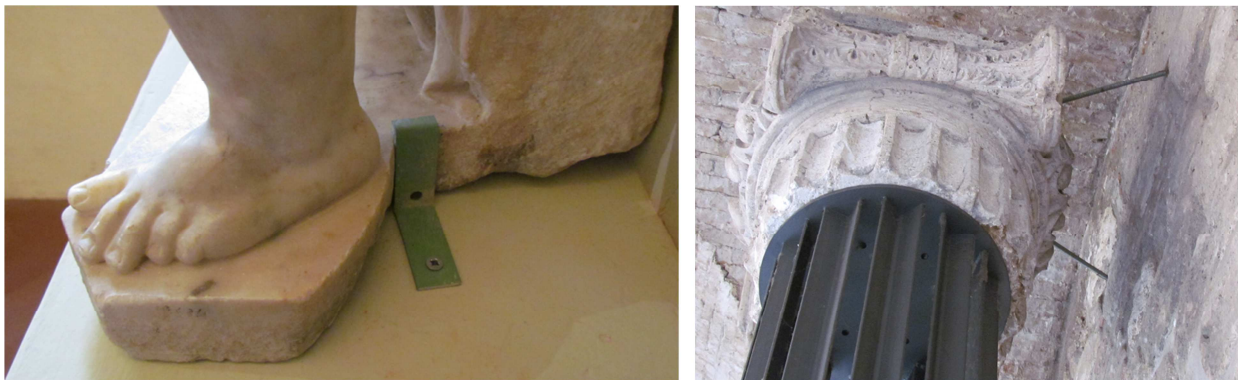
Figure 5.10 Examples of seismic risk mitigation for art object by means of anchoring systems
