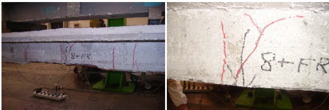
Fig. 4.40: Pictures of the crack pattern of the concrete web near the mid-span of the beam 101
