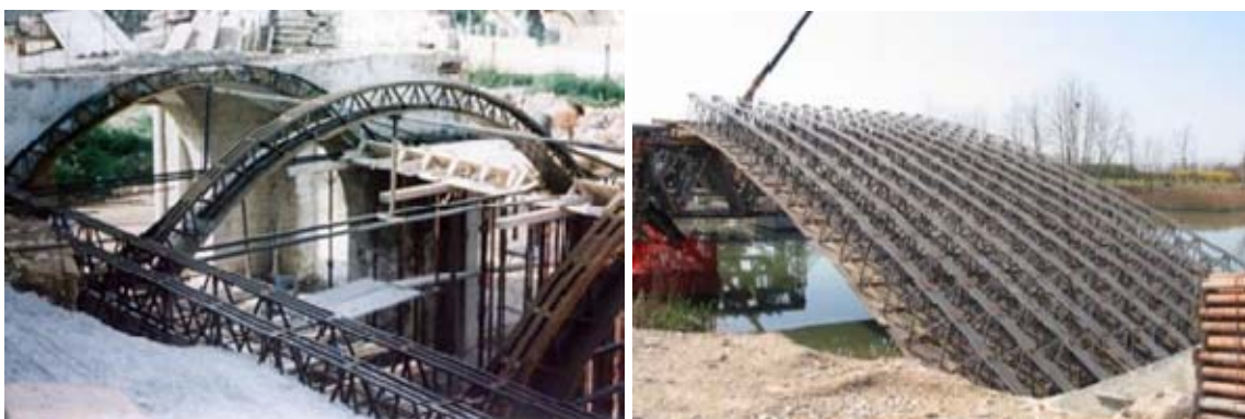
Fig. 1.7: Curved and arch steel truss examples (Italy)
