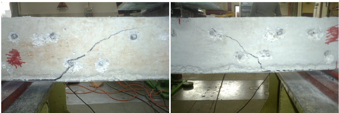
Fig. 4.20: Pictures of the beams 4 after the collapse
