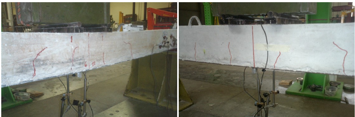
Fig. 4.16: Pictures of the beams 3 after the collapse
