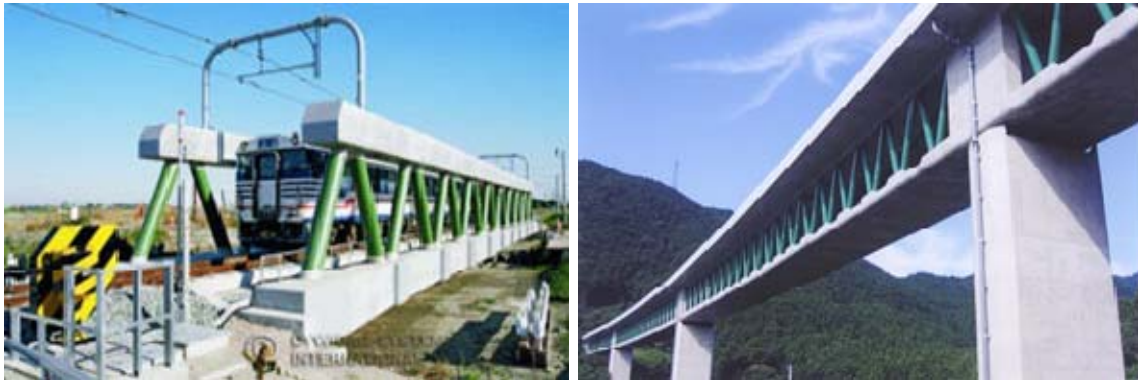
Fig. 1.1: Composite steel and concrete truss bridges: Yamaguragawa Bridge (Japan) and Kinogawa Bridge (Japan)
