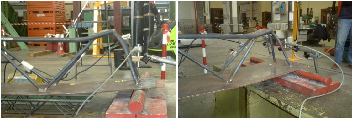
Fig. 4.9: Pictures of the trusses 1 after the collapse
