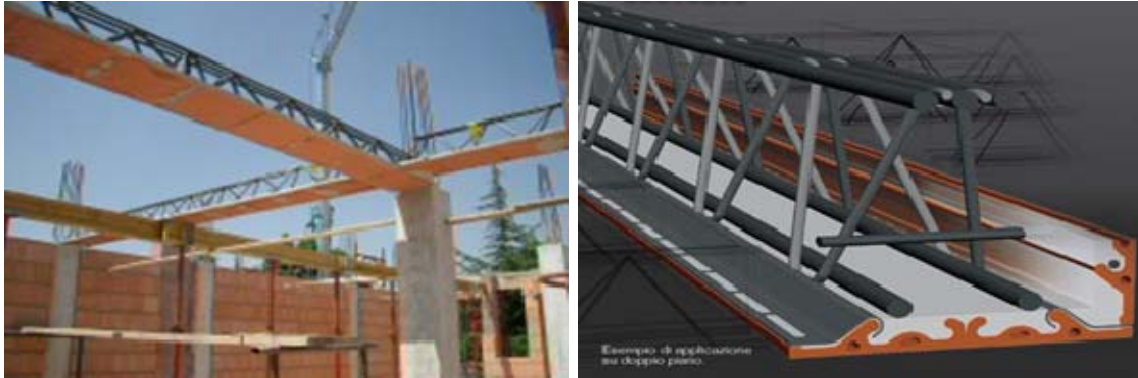
Fig. 1.5: Tecnostrutture's composite steel truss and concrete beams with the inferior clay tile (Italy)
