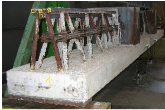
Fig. 4.57: particular view of a truss beam head
