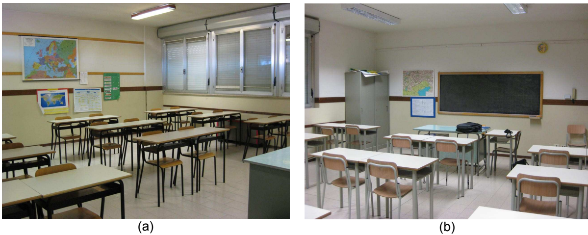
Figure 4.18 – Lighting appearance with the old luminaries (a) and with the new ones (b).
