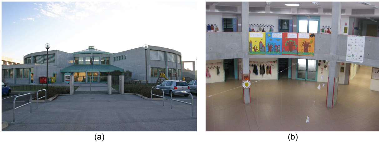
Figure 6.4 – School exterior (a); the atrium (b)
