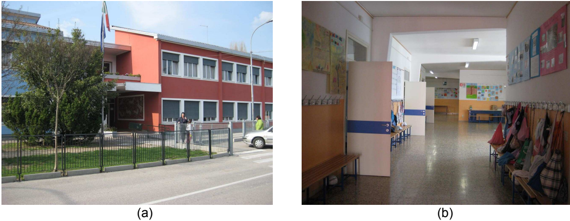
Figure 6.9 – School exterior (a); the aisle (b)
