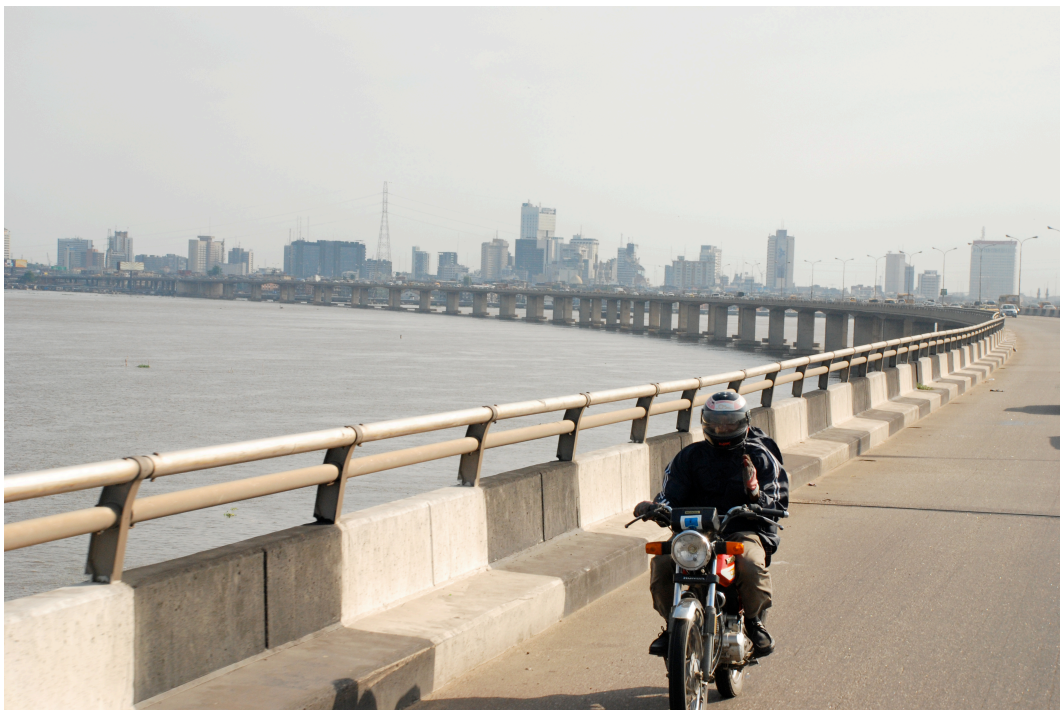
Figure 14. Third mainland bridge. Lagos.
