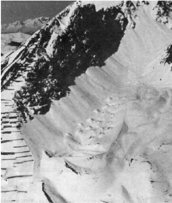
Fig. 4.96 – Active and passive defence structures at Davos, Canton of Grisons, Switzerland [McClung & Schaerer, 1996].
