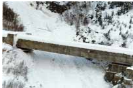
Fig. 4.60 – Direct protection structures: a) building reinforcement techniques; b) reinforcement techniques for structures; c) protecting wedges or splitters; d) roofing; e) avalanche tunnels [ http://cagem.bayindirlik.gov.tr ; Somnavilla, 2006; McClung & Schaerer, 1996].
