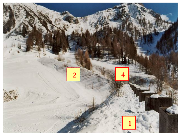
Deflecting dams 2, 4 and catching dam 1 [photo by Moro, 2008].
