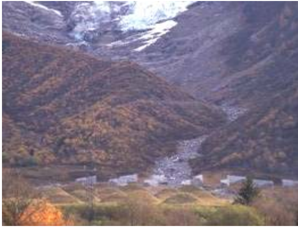
Retarding tooth-shaped structures I and vertical walls [http://cemadoc.cemagref.fr].
