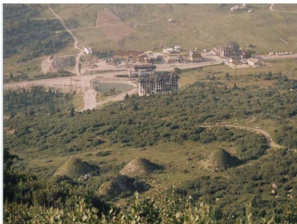
Retarding cone-shaped structures [photo by Bezzi, 2004].
