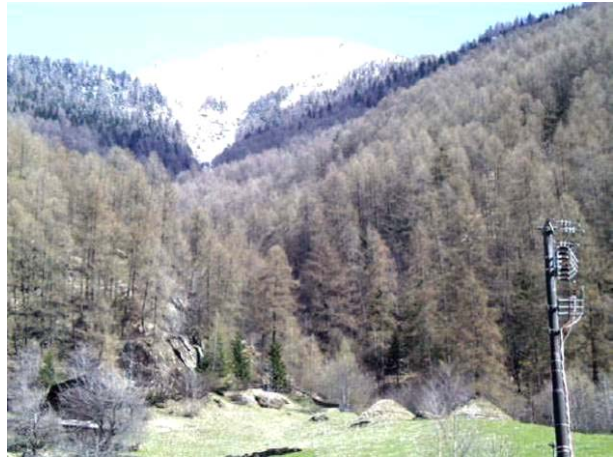
Retarding cone-shaped structures [photo by Trento Province].
