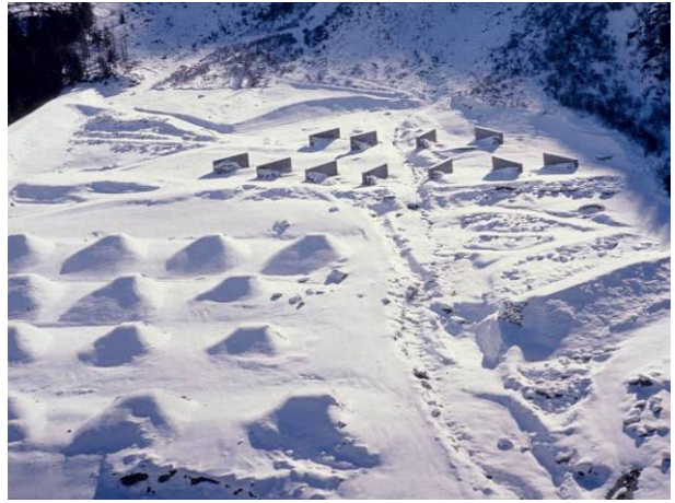
Retarding tooth-shaped structures I and vertical walls [http://cemadoc.cemagref.fr].
