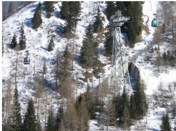
Protecting wedge [photo by Tomaselli, 2007].
