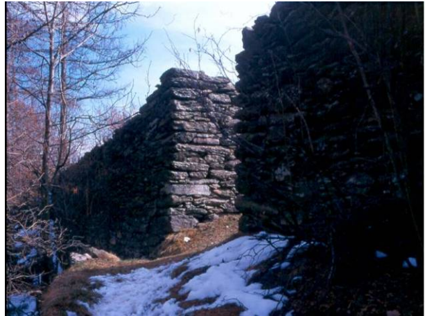
Catching dam [photo by Municipality of Finestrelle].
