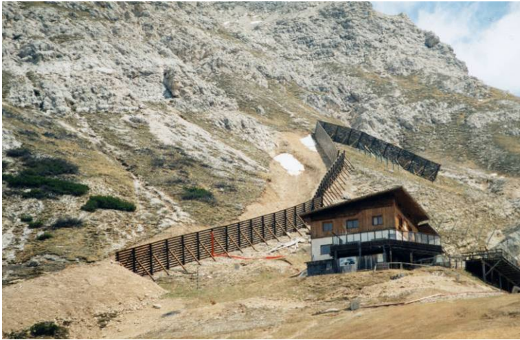
Catching dam and protecting wedge [photo by Tomaselli, 2007].
