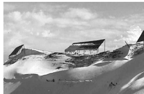
Fig. 4.10 – Snow fences or redistribution structures: a) wind baffles; b) snow wind fences; c) wind panels; d) jet-roof [http://cagem.bayindirlik.gov.tr; http://www.arpa.veneto.it/csvdi; McClung & Schaerer, 1996].
