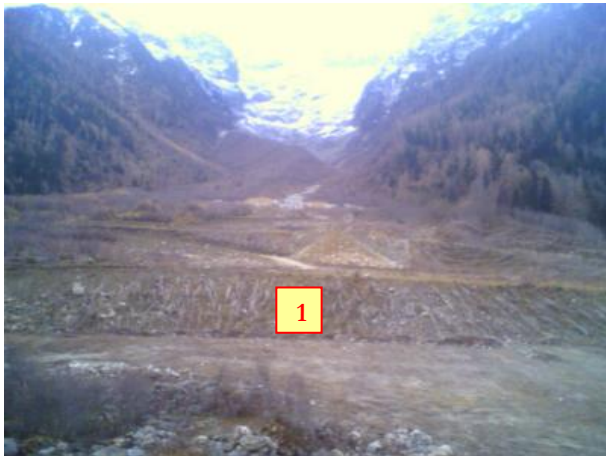
Catching dam 1 [ http://cemadoc.cemagref.fr ].
