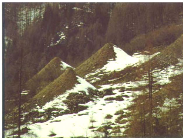
Retarding cone-shaped structures [photo by Trento Province].
