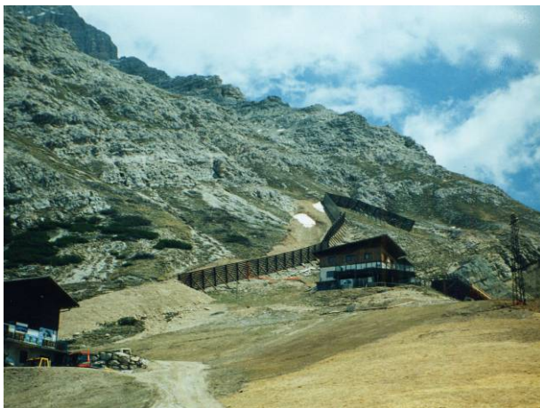
Catching dam and protecting wedge [photo by Tomaselli, 2007].
