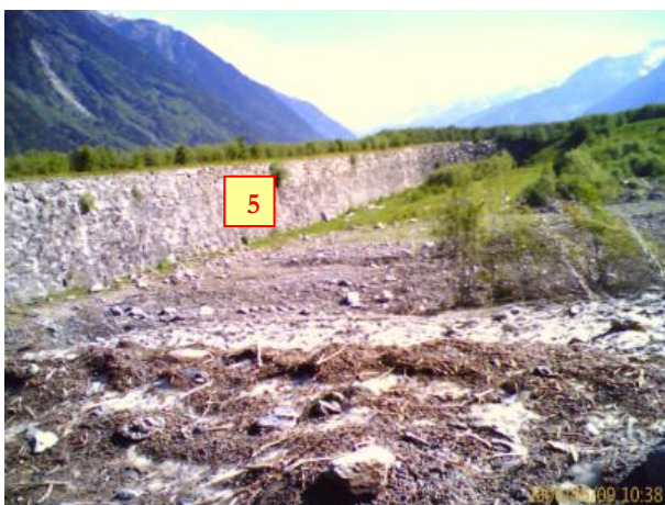
Deflecting dam 5 [http://cemadoc.cemagref.fr].
