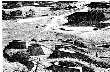
Fig. 4.33 – Retarding or braking mounds: a) retarding cone-shaped structures; b) retarding tooth-shaped structures [ http://cagem.bayindirlik.gov.tr ; Frutiger & Martinelli, 1983].
