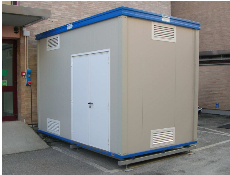
Figure J.1. The container in the courtyard of the Department of Information Engineering (DEI) of the University of Padova. Its surface is equal to 9.6 m 2 . It is connected to the department electrical grid ( P_{e,M} = 20 kW) and to the department Local Area Network (LAN).
