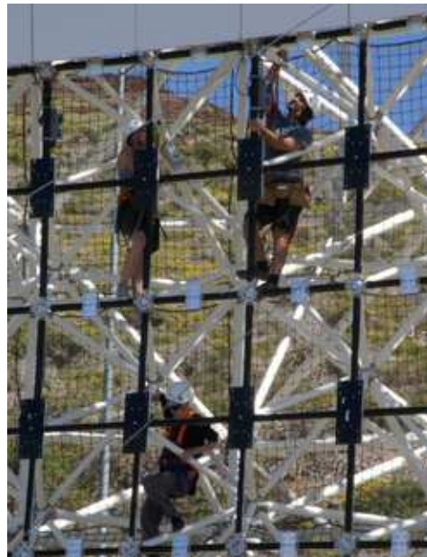
Figure 3.5: MAGIC spaceframe structure
