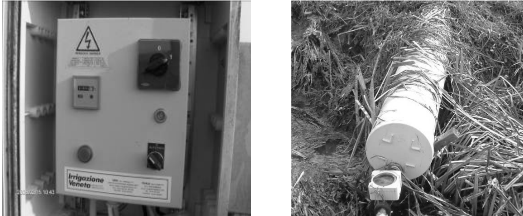
Figure 8 – Flow meter at the inlet and at the outlet of the SFW
