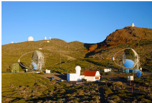
Figure 3.28: Image of the MAGIC stereo system. Close to the MAGIC I (left) and the MAGIC II (right) telescope, which are spaced by a distance of \sim 85 m, the counting house (center). Credit R. Wagner/MPI Munich.
