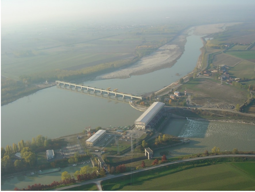
Figure 1.1: Aerial view of the Isola Serafini run-of-river power plant (Piacenza, Italy).
