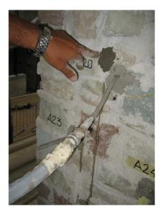
Figure 2.7: Grout injection.
