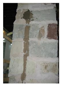
Figure 2.8: Grout leak from a masonry crack.
