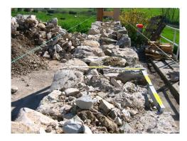
Figure 2.13: Detail of the cross section of the wall.
