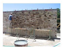
Figure 2.17: Injecting lime grout.
