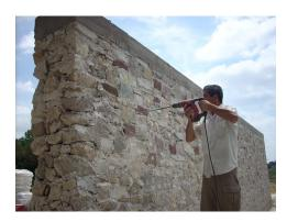
Figure 2.16: Drilling holes in the wall.
